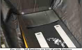
Fig 102 - Tail flashing on top of side flashing
