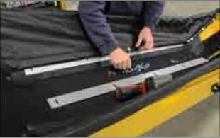
Fig 94 - Stainless steel flat bar to hold side flashing
