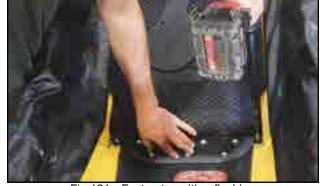
Fig 101 - Fasten transition flashing
