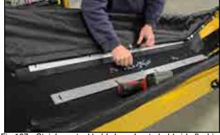
Fig 107 - Stainless steel hold-down bar to hold side flashing
