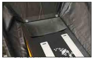
Fig 92 - Tail flashing on top of side flashing
