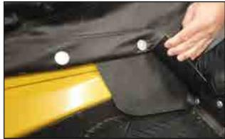
Fig 106 - Flashing fastened along transition
