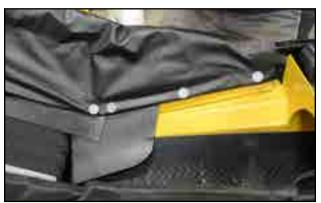
Fig 93 - Transition corner flashing in place
