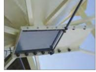
Rack-n-Pinion slide gate assembly Premium Rack-n-Pinion slide gate assembly with crank; also available in stainless steel.
