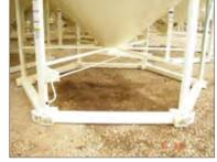
**Skid Foundation** Skid foundations are available for most bins.
