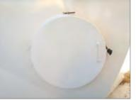
Roof Manhole Access hole in top cone.
