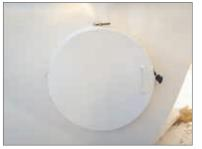
Roof Manhole Access hole in top cone.
