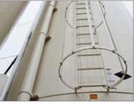
Ladder Cage (Sidewall) Safety enclosure for added security. Roof handrail also available.
