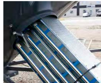
Slide Retro Rocket through manhole
